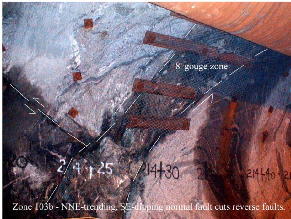
**Figure 7** – The geology of this disturbed interval (Station 214+30, left wall) is dominated by a major NNE-trending SE-dipping normal fault exposing a 3m thickness of clay-rich crush breccia. The NNE fault of Group D displaces older low-angle reverse faults (Group A) in both the footwall and hanging wall blocks of the fault. Fault splays of various orientation and offset sense are found adjacent to the NNE-fault. [Image by C. Merguerian, 18 November 1999.]
