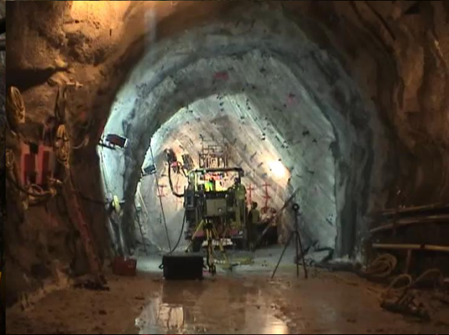
Harlem River Tunnel - 2009
