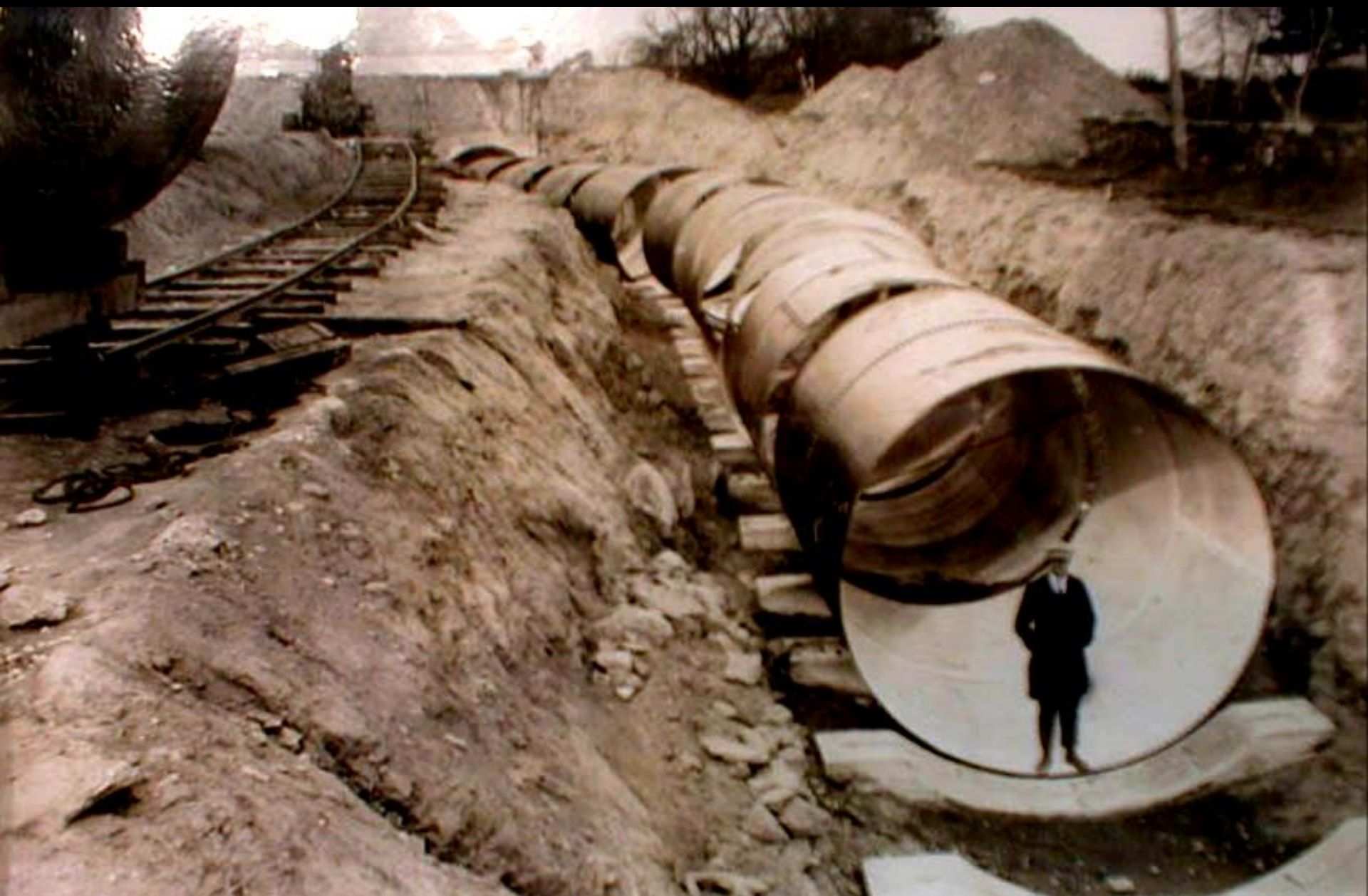
Cut and Cover Tunnel, Catskill Aqueduct
