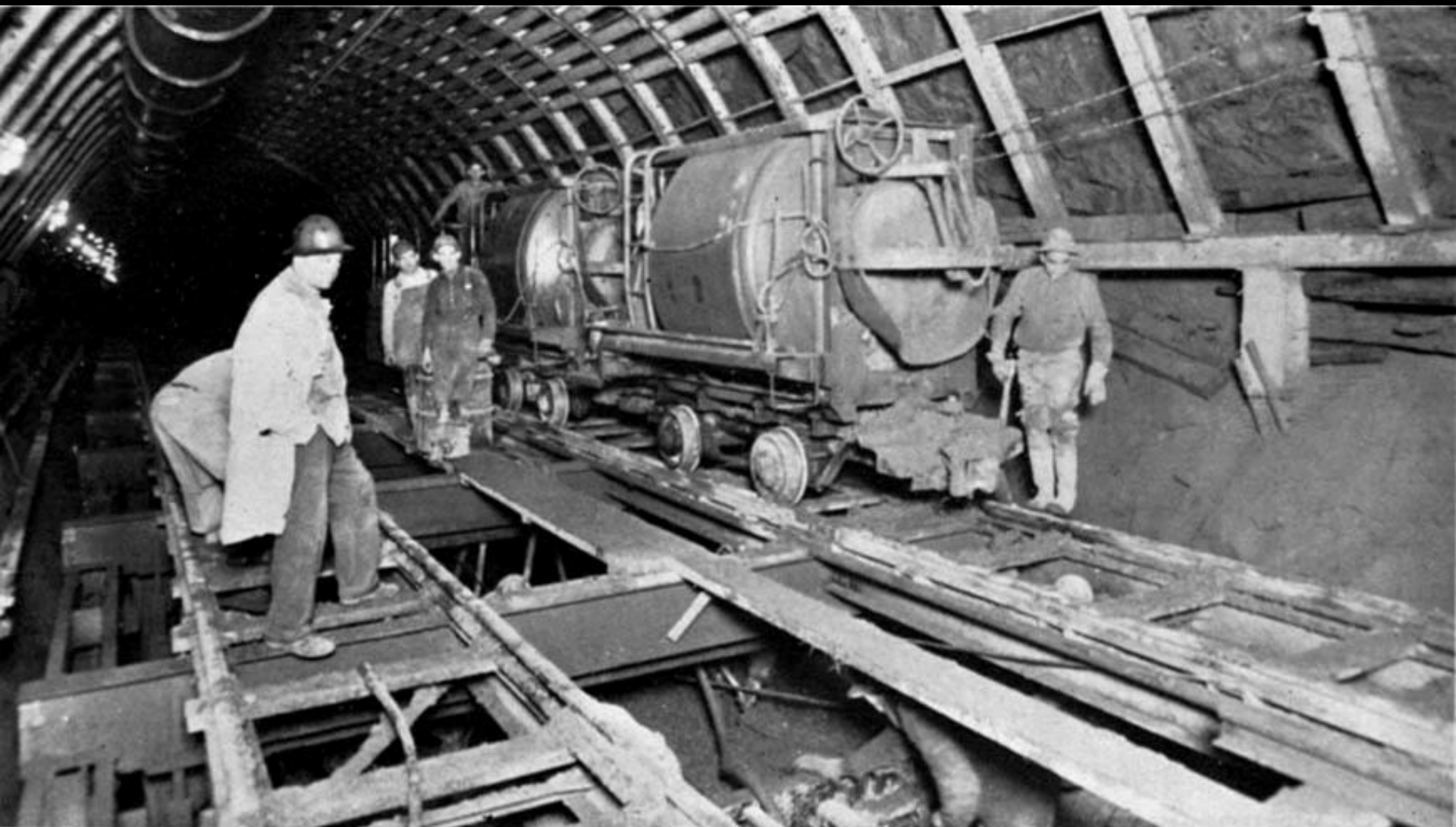
Invert Pour, Delaware Aqueduct, Kensico Hill View Tunnel
