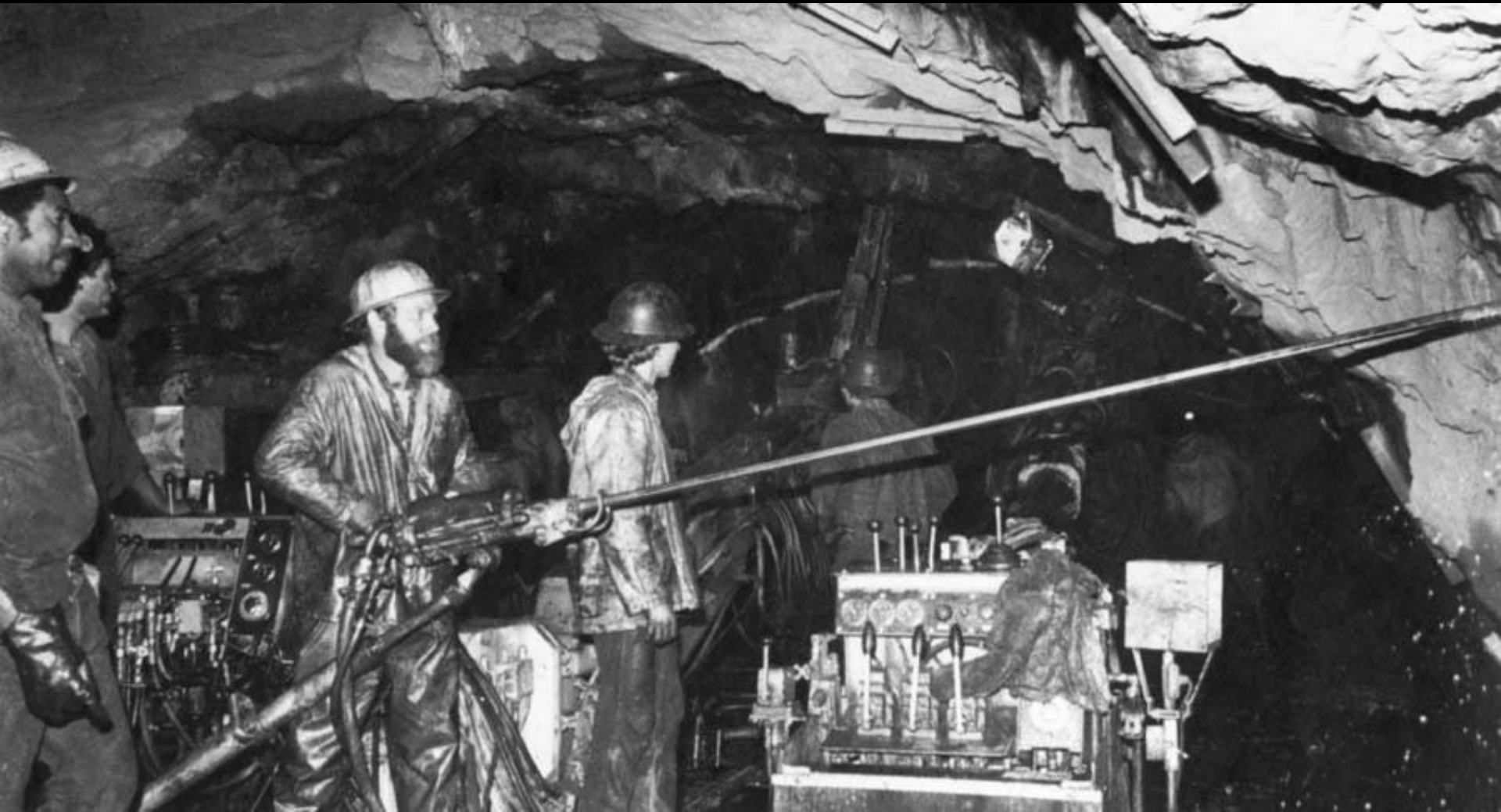
City Tunnel #3, Stage 1 – Drill and Blast Technology
